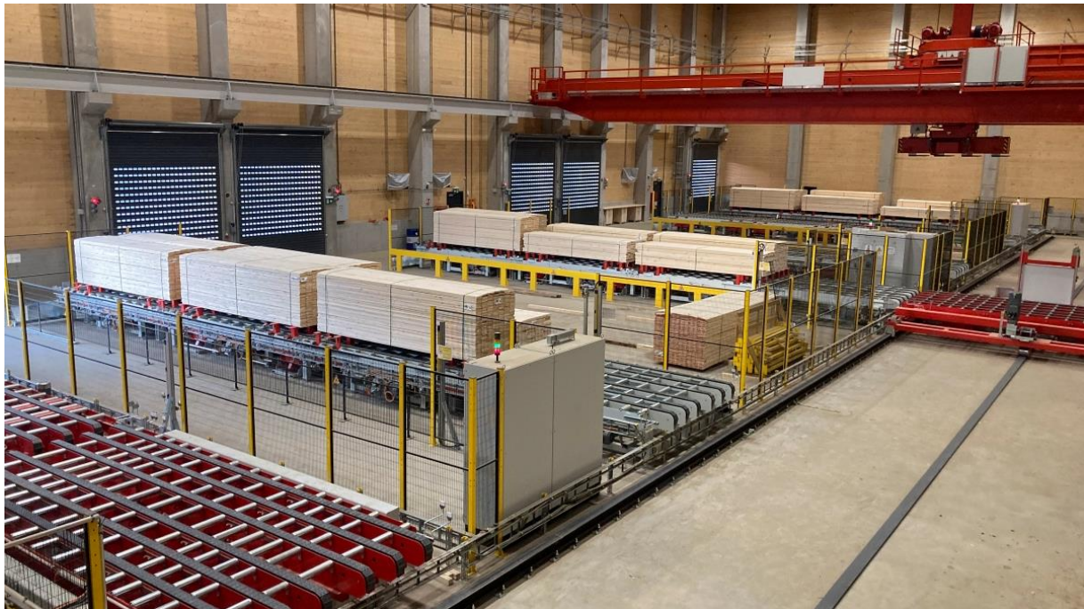
Illustration 2 Semi-automatic trailer loading zone with modular belt conveyors and lifting rams for up to 12 tons
